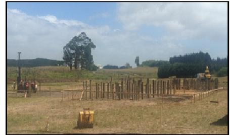
The first order of business for the contractors were the trenches for the common services and preparing the sites for the piles of the whare. The contractors then started laying the floors, followed by the erection of the prefabricated framework for the 5 whare. All of the rooftops are now on and the aluminium joinery has been fitted into place, currently the builders are working on lining the exterior and interior of the whare.
